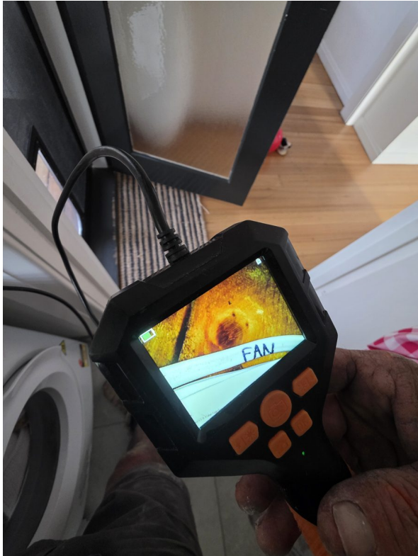
5. Camera inspection of internal wall framing (laundry)
