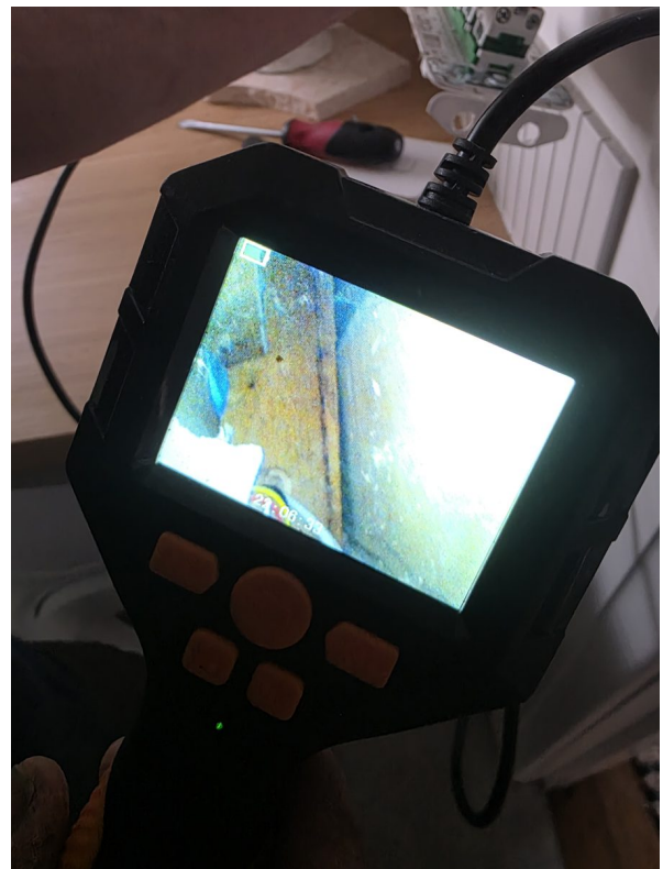
8. Camera inspection through power point opening
