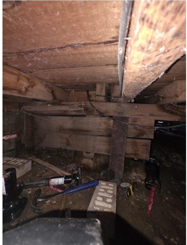
2. During works: floor propped and affected timber removed
