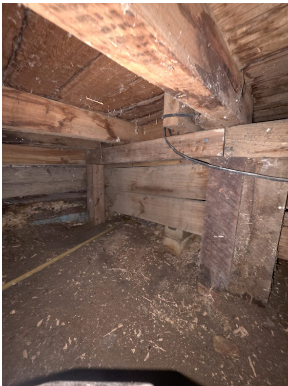
3. After: new bearer timber installed
