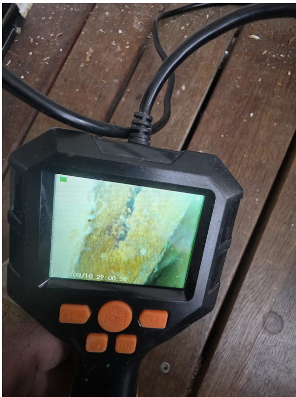
7. Camera view of wall frame timber
