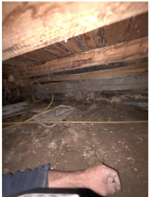
4. Subfloor inspection of surrounding bearers, joists and stumps
