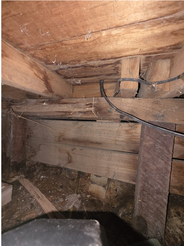
1. Before: original bearer where termite activity may have been present
